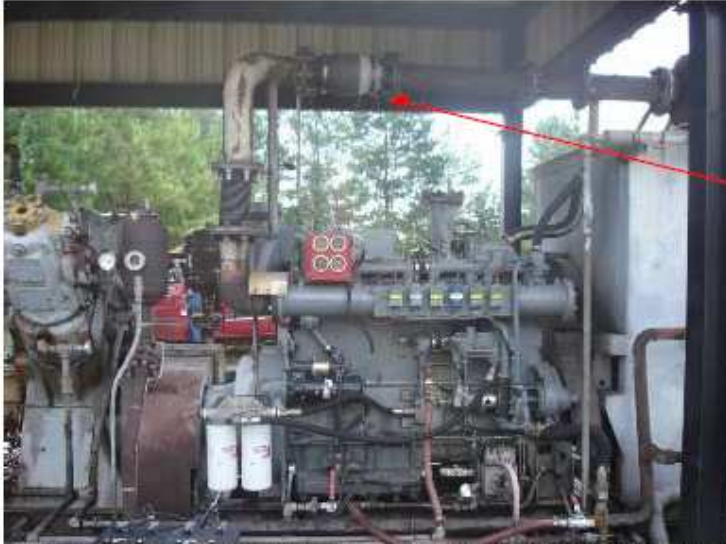
Figure 1. BP Findlay Compressor Station with Catalyst Installation.
